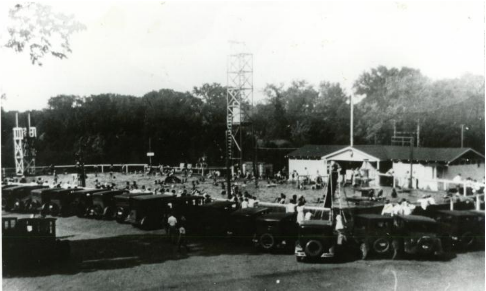
Carr's Pool, built by R.E.(Dad) Carr in 1926. Note the diving platform at the north end of the pool and the large fountain in the pool's south end where children gathered. The tower at the left of the old bath house supported the pressure tank when Carr relied on his own well. In this photo, the diving platform had been extended to a height of 50 feet. On two occasions, Fred Poole and Bill McLaughlin made high dives from that tower adding a real thrill to swimming and diving exhibitions. When McLaughlin scraped the bottom, he was not seriously injured, but Dad Carr said, "No more high dives!"
